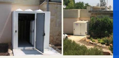
Experienced from past missile strikes, the Council set a requirement that the power source suit a protected space within a bomb shelter; this prerequisite established strict restrictions in terms of the generator's size, noise and emissions, limitations which standard diesel generator backup solutions could not meet.
